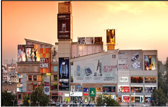
Fig. 14. DLF City Centre, Gurgaon.
